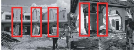
Fig. 3 - Partially collapsed structures after the 2004 Tsunami in Sri Lanka
