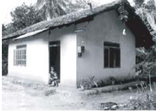
Fig. 1 – Traditional house being rebuilt in Sri Lanka
