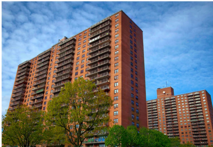
Nelson Management's Atlantic Plaza Towers
